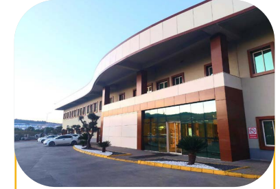
Gaziemir Facility (Aegean Free Zone)
